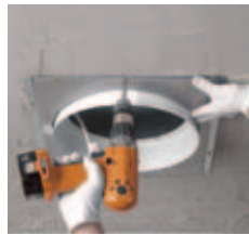
2 install Gypkit for downnut in front of the Downnut conbox
