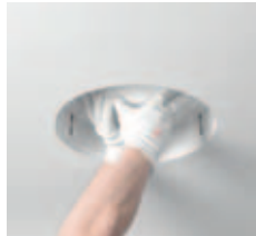
6 lock the fixture to the housing by turning clockwise on the screws
